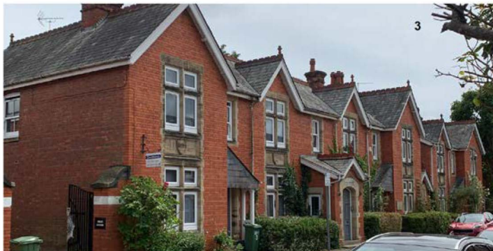
Images 3 - 1 - 4 Peel House and Bailey House, Bartelot Road "Former police station buildings. Peel House is two storey with four gables fronting the road, and central porch and door. West Sussex County shield carved in stone between ground and first floor. Brick with stone dressings and a slate roof. Bailey House built to similar designs, however of a smaller street front with two gables. In use as a police station between 1894 and 1973. Now used as offices. Gates to rear yard display the Centenary 1994 police badge. Built 1884." Image 1 - Christian Life Church East Street "Previously the Pentecostal church and originally the Primitive Methodist church. Brick built, with 3 bays, the central one over the door below. Decorative terracotta panels with pediments and finials. Plaster decorative panels. c.1891." Image 2 - 51 and 53 East Street "51 East Street is a 2 and a half storey Victorian brick building, with projecting bay window at first floor and a quality traditional shop front at ground floor. It forms a group with number 53, of which the most prominent feature is the corner tower at first and second floor. c.1890" Text taken from the 2011 Horsham Town Local List
