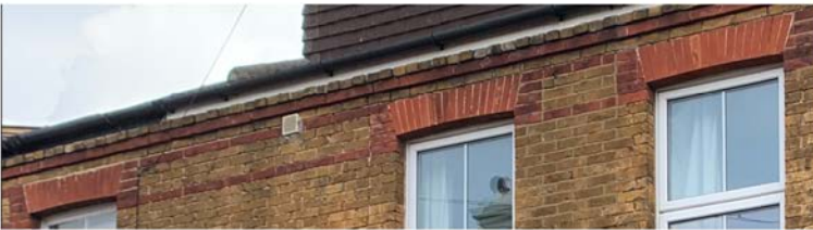
Stretcher bond with decorative soldier course and window details.
