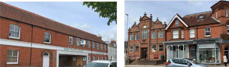
Commercial properties within Barttelot Road
